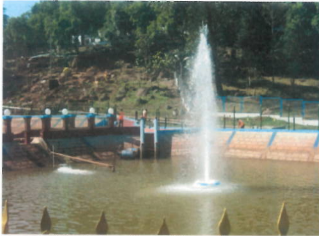
Rain water harvesting pond Noamundi
