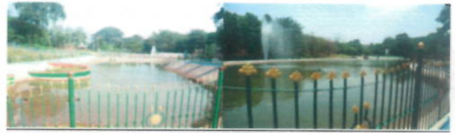
RWH structure for ground water augmentation in the area
