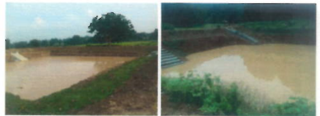
Newly constructed ponds in surrounding villages
