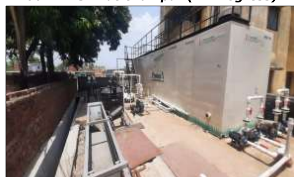
100 KLD STP at Chainpur (In Progress)
