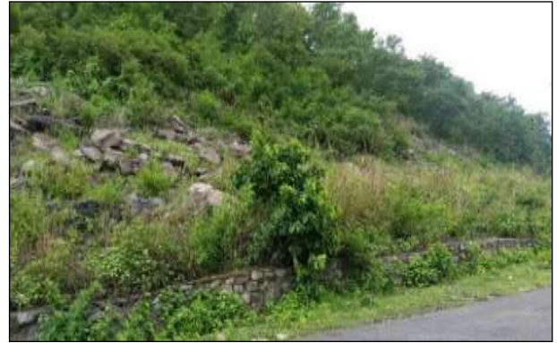
Toe walls on dumps
