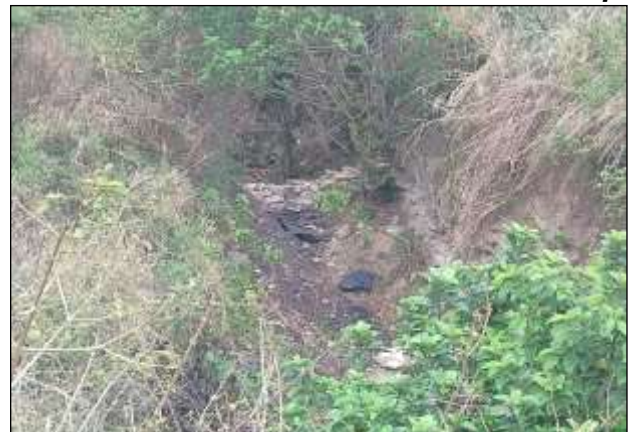
Catch Drains with check dam at the toe of dumps
