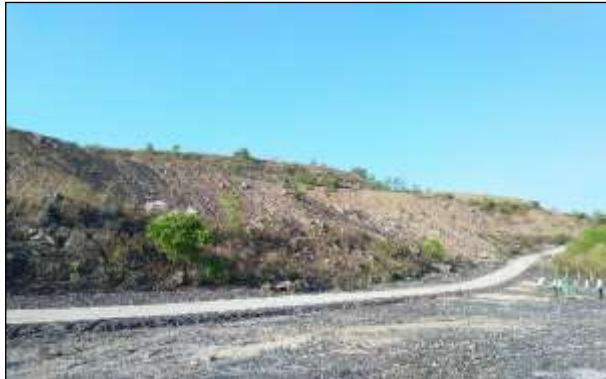
Soil & grass Spreading on dump slope
