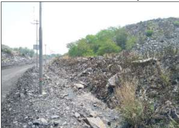
Catch Drains at the toe of dumps
