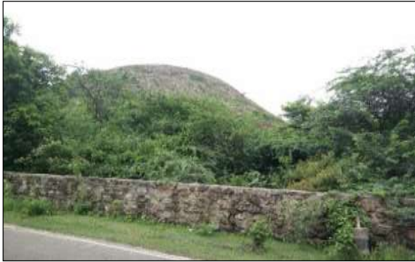
Toe walls on dumps
