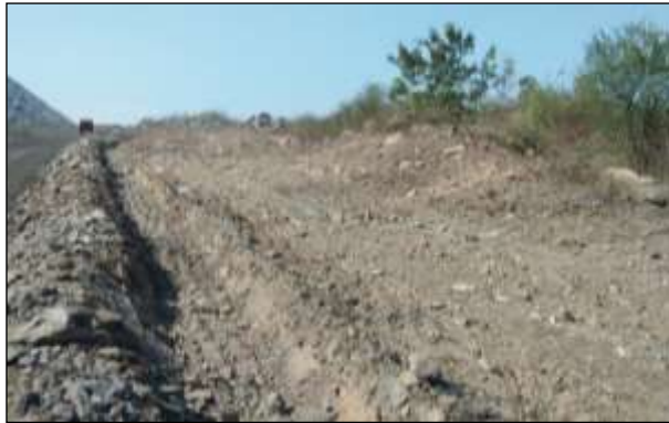
Maintained catch drain of Topsoil Dump
