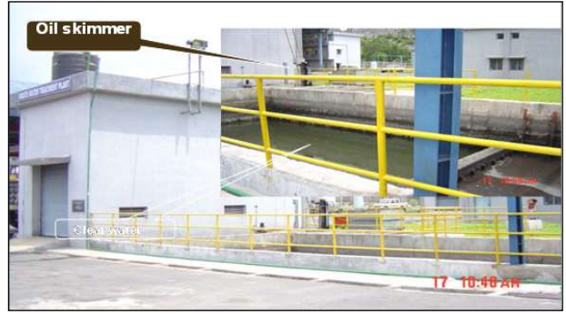
Oil & Grease trap at mines
