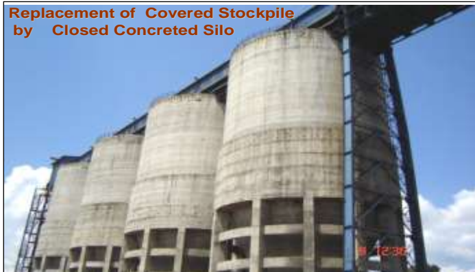
Concrete silos for material storage
