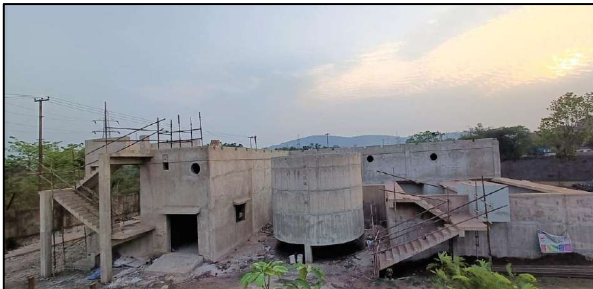
EFFLUENT TREATMENT PLANT (ETP)-30 M3/HR UNDER CONSTRUCTION
