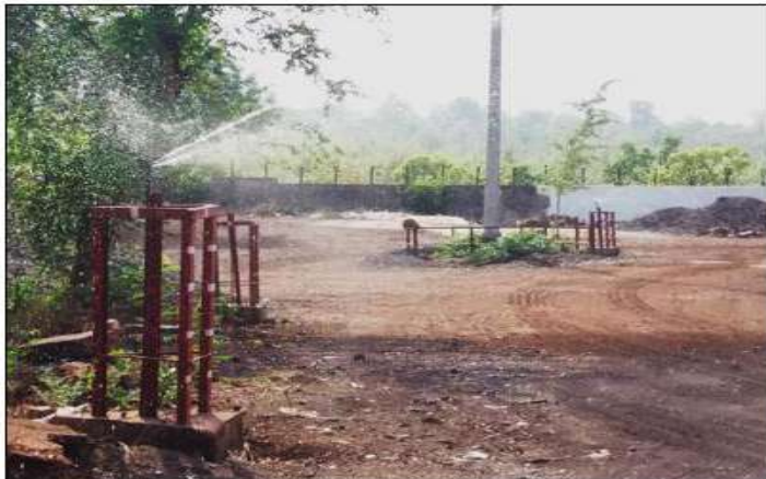
Auto Sprinkling of Water for Dust Suppression
