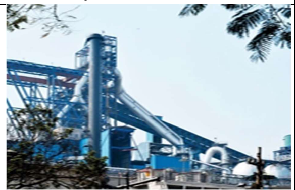
High Efficiency BF with high Top Pressure, Stove Waste Heat Recovery, TRT, Cast House Slag Granulation
