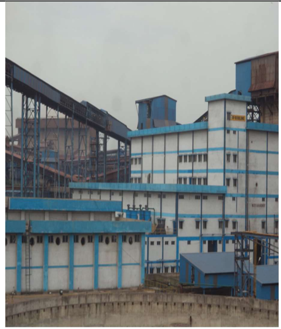
Reverse Osmosis Building
