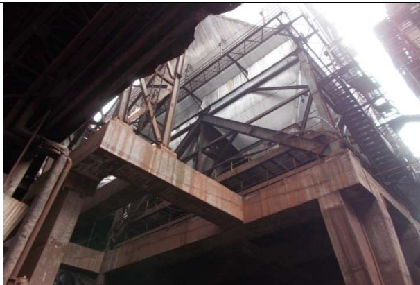
Sinter Plant 2 Refurbished ESP
