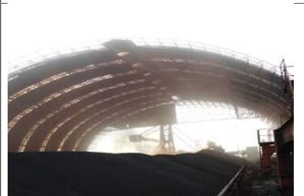
Covered Shed for Coal and Pellet
