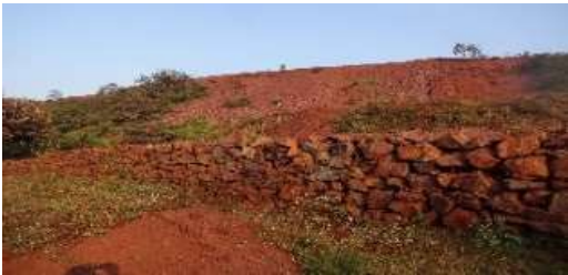
Toe Wall & Garland Drains for Runoff Management
