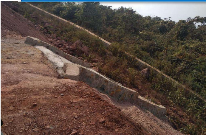
Toe Wall & Garland Drains for Runoff Management
