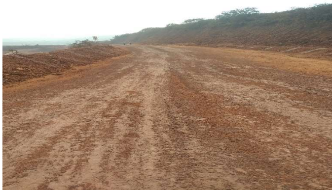
Mine Haul Road
