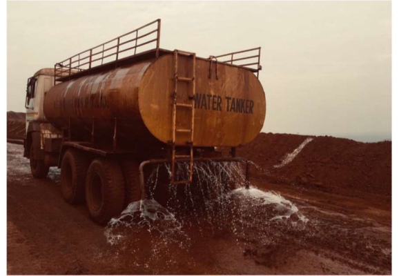
Grader for Haul Road
