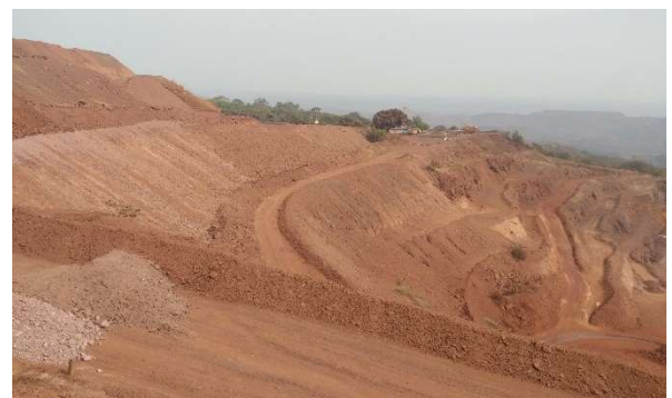
Benches along Dump Slope
