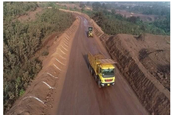
Mine Haul Road with Safety Berms
