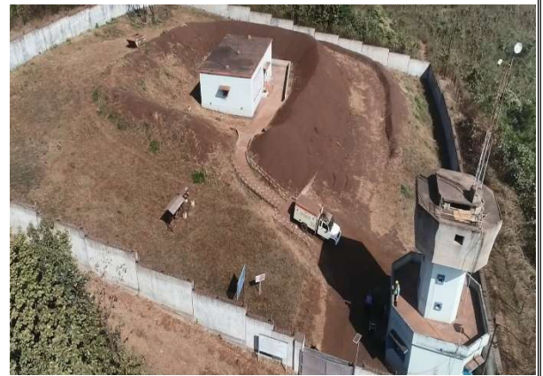
Central Magazine for Storage of Explosive
