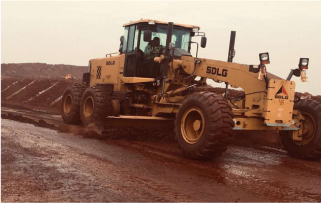
Grader for Haul Road
