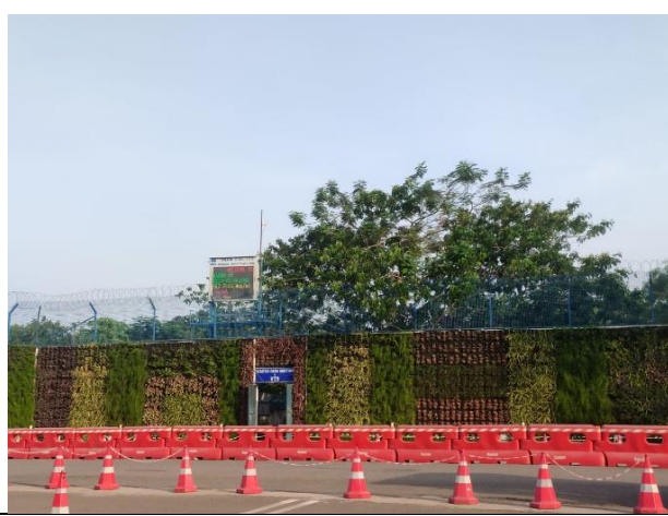
Vertical garden and digital display board at Main gate
