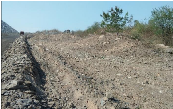
Maintained catch drain of Top Soil Dump
