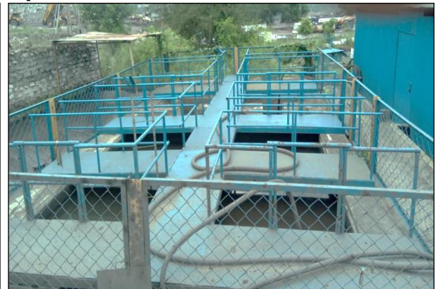
Oil & Grease trap at mines
