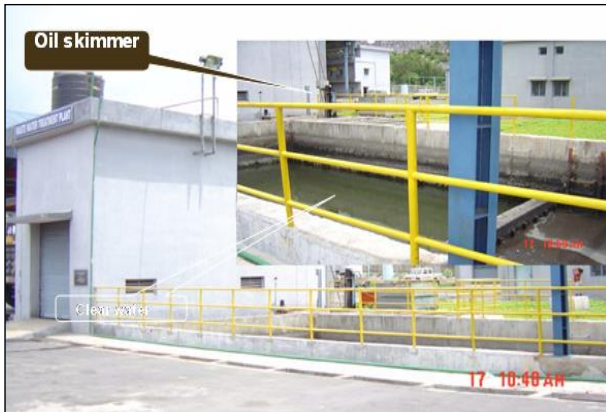
Oil & Grease trap at mines
