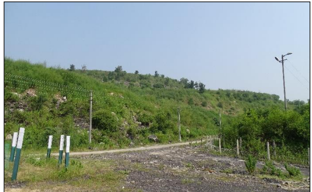
Grassing and Plantation on dump slope
