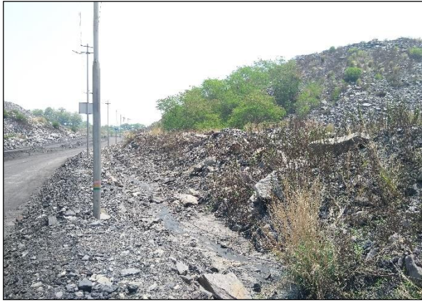
Catch Drains at the toe of dumps
