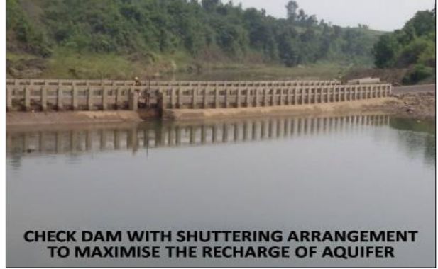
Check Dam to increase ground water recharge
