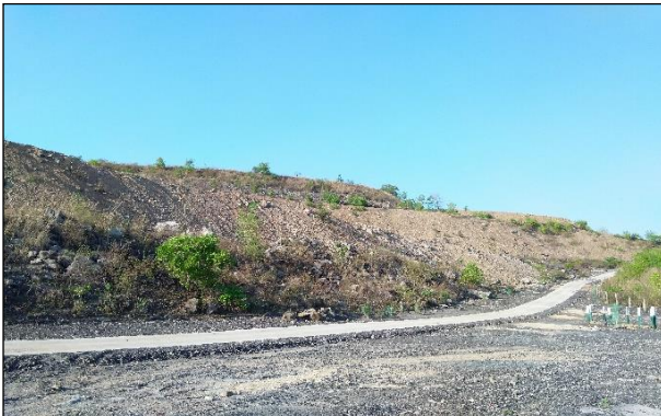
Soil & grass Spreading on dump slope
