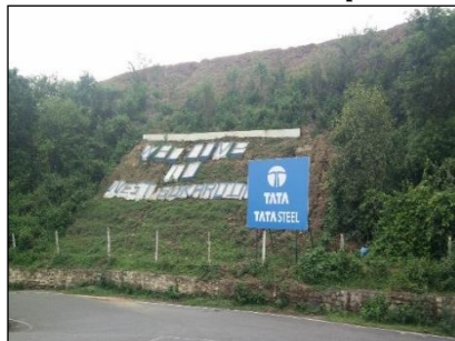
Toe walls on dumps
