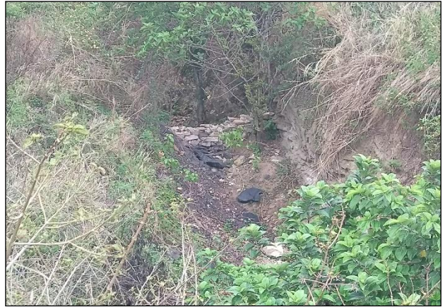
Catch Drains with check dam at the toe of dumps
