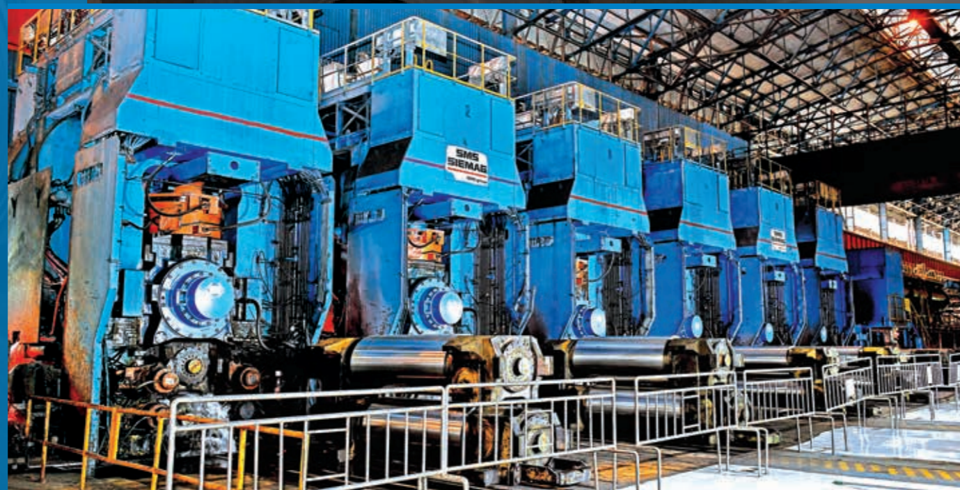
Thin slab caster and rolling facility at Jamshedpur Steel Works
