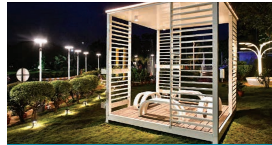
Fibre Reinforced Polymer (FRP) structure at Jamshedpur Steel Works
