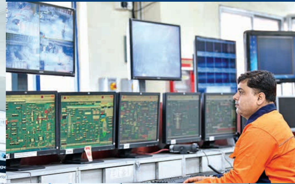
Control Room, Jamshedpur Steel Works
