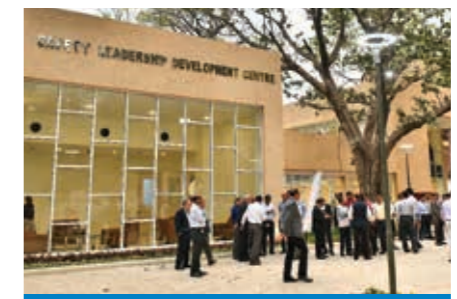
Suraksha Kendra, Jamshedpur Steel Works
