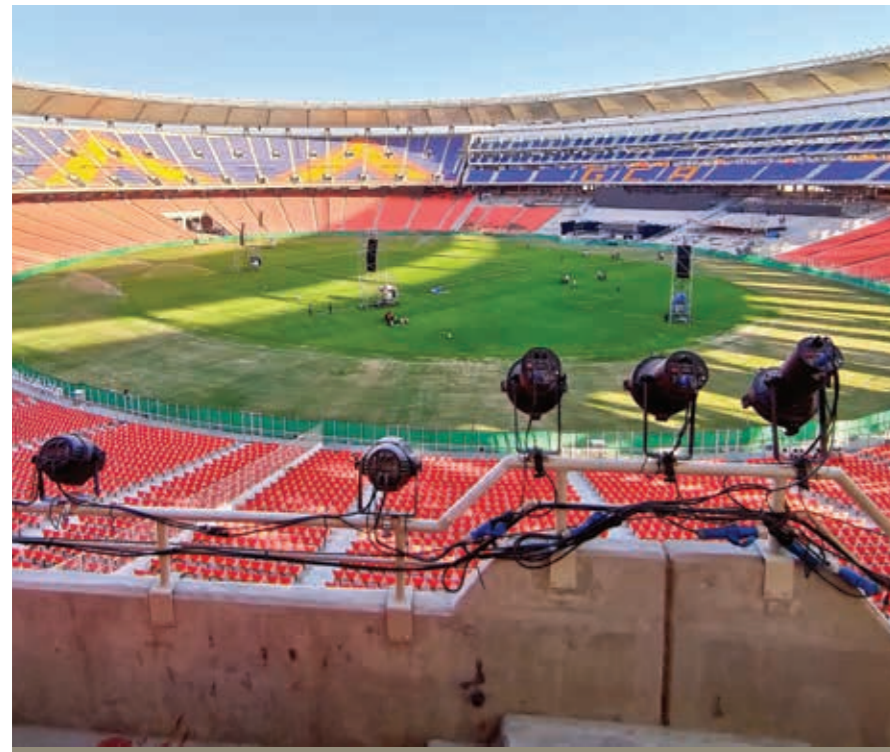
Sardar Patel Stadium, Ahmedabad — We are proud to be the major steel supplier to this world-class project, having supplied 75% of the rebars, besides 41,000 couplers and 8,400 threads to expedite the completion.
