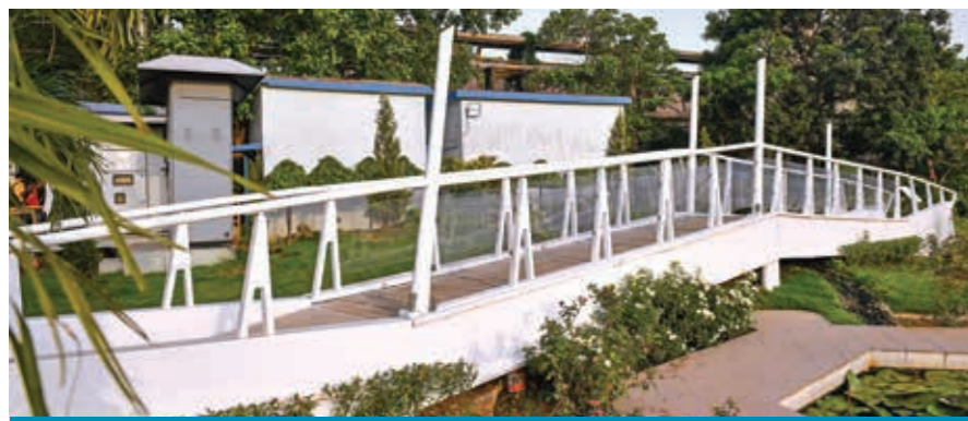
Fibre Reinforced Polymer (FRP) bridge at Jamshedpur Steel Works
