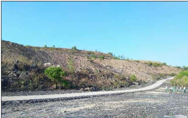
Soil & grass Spreading on dump slope
