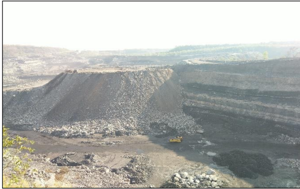
Back filling of quarry by Over Burden
