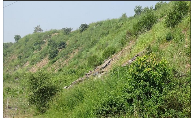
Grassing and Plantation on dump slope
