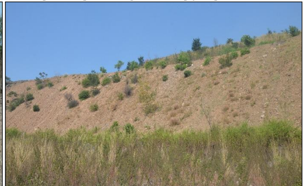
Top Soil spreading on dump for plantation
