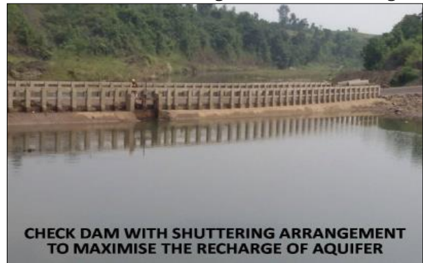
Check Dam to increase ground water recharge
