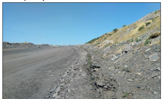
Catch Drains at the toe of dumps
