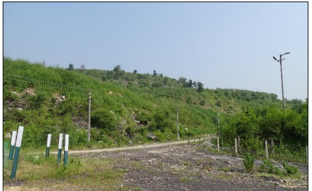
Grassing and Plantation on dump slope
