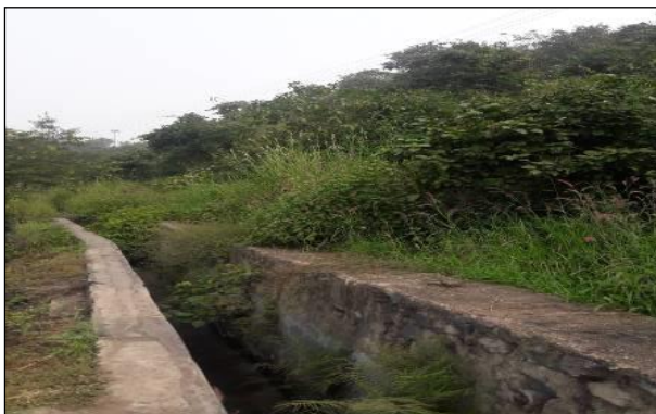
Catch Drains at the toe of dumps
