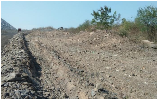
Maintained catch drain of Top Soil Dump
