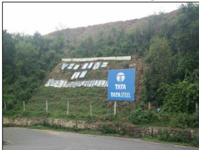
Toe walls on dumps
