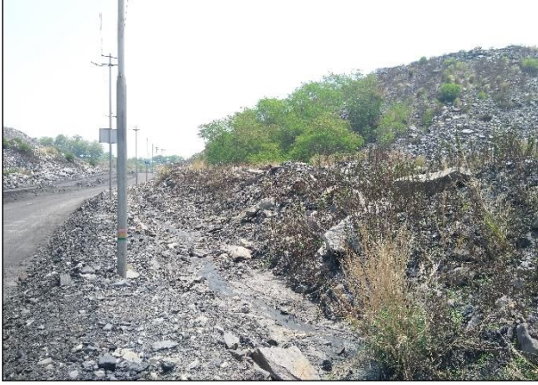
Catch Drains at the toe of dumps
