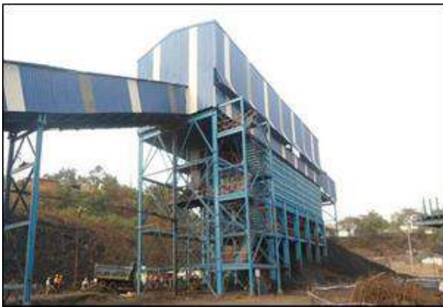
Coal transport by conveyor belt
