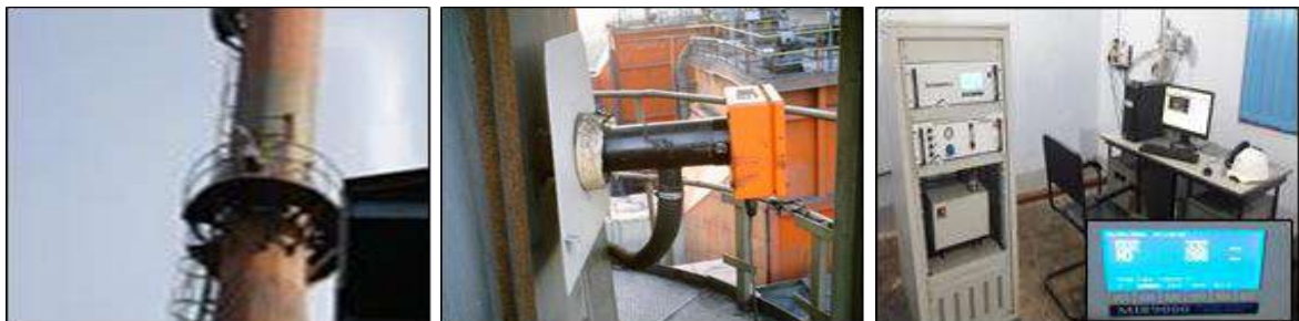
Continuous Emission Monitoring for Power House for PM, Sox & NOx data
