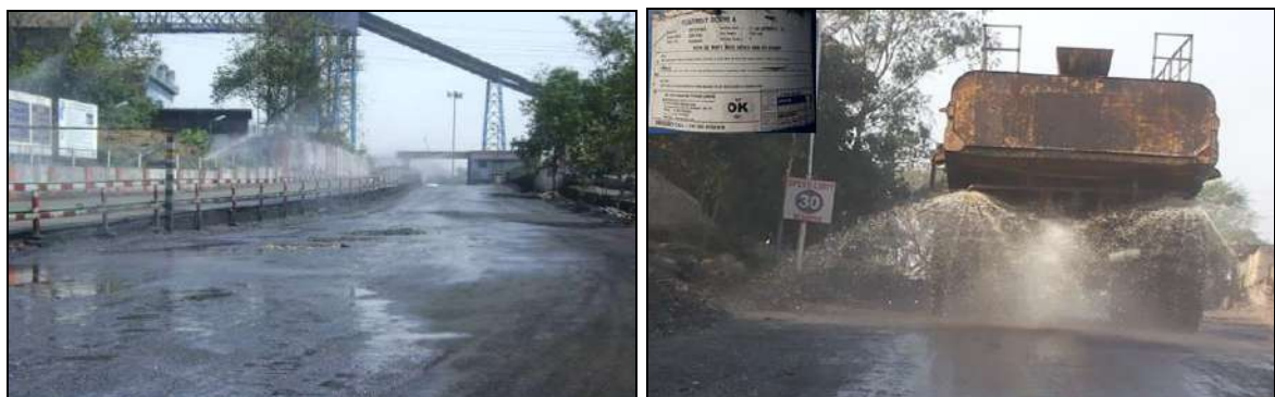
Fixed and mobile water suppression system
