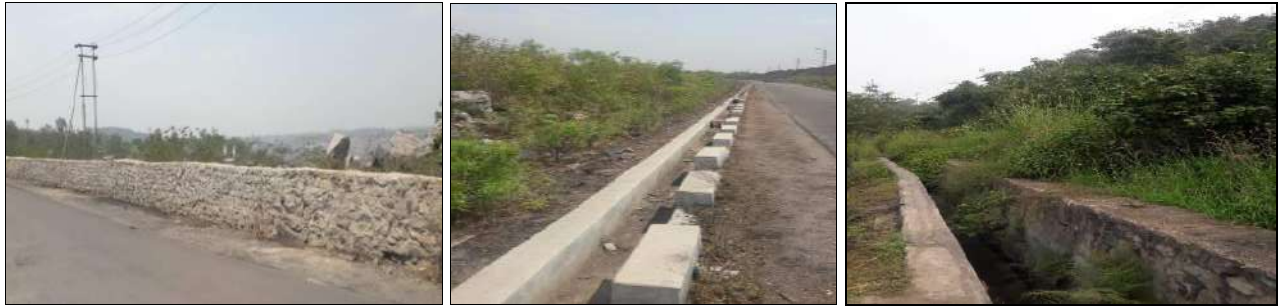
Toe wall & garland drain in the area
