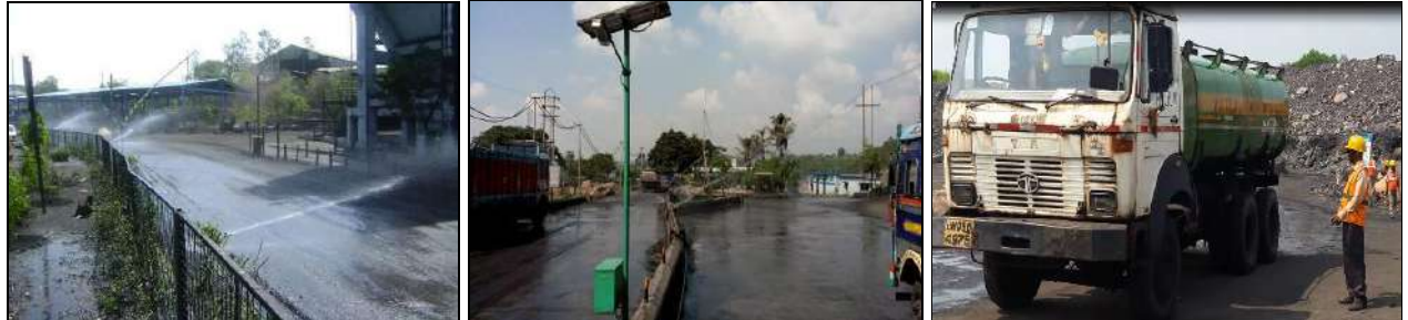
Use of Fixed & mobile water sprinklers in area
