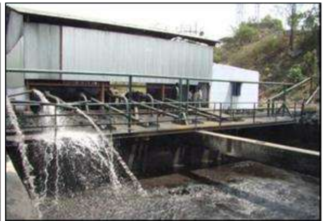
Effluent recycling in washery
