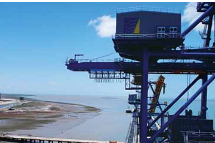
Top: LD #3 plant under construction, Jamshedpur. Middle: 'I' Blast Furnace under construction, Jamshedpur. Bottom: Construction in progress at Dhamra Port.
