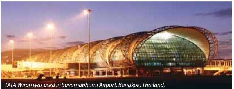
TATA Wiron was used in Suvarnabhumi Airport, Bangkok, Thailand.
