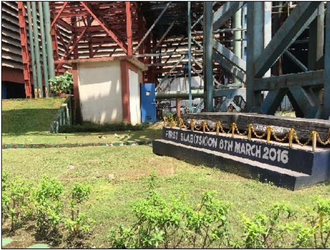
First Slab casted in TSK
