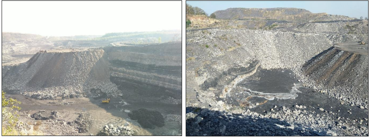
Back filling of quarry by Over Burden
