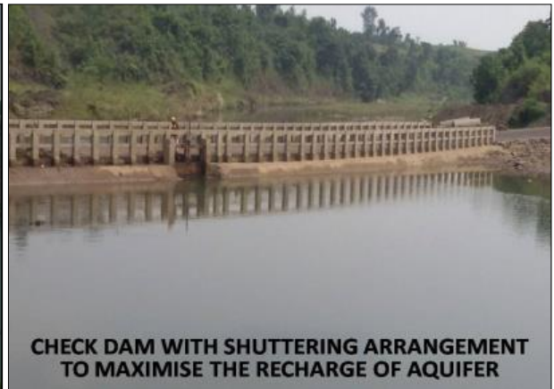
Abandoned Mine pit converted into RWH pond Check Dam to increase ground water recharge
