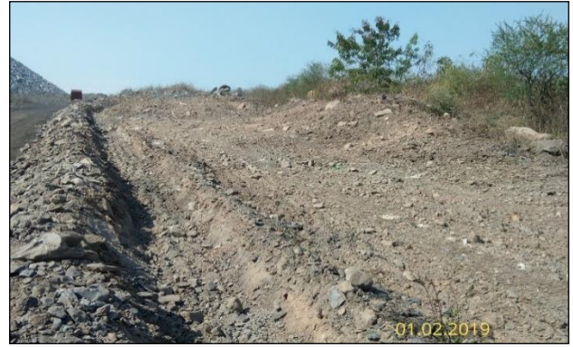
Maintained catch drain of Top Soil Dump
