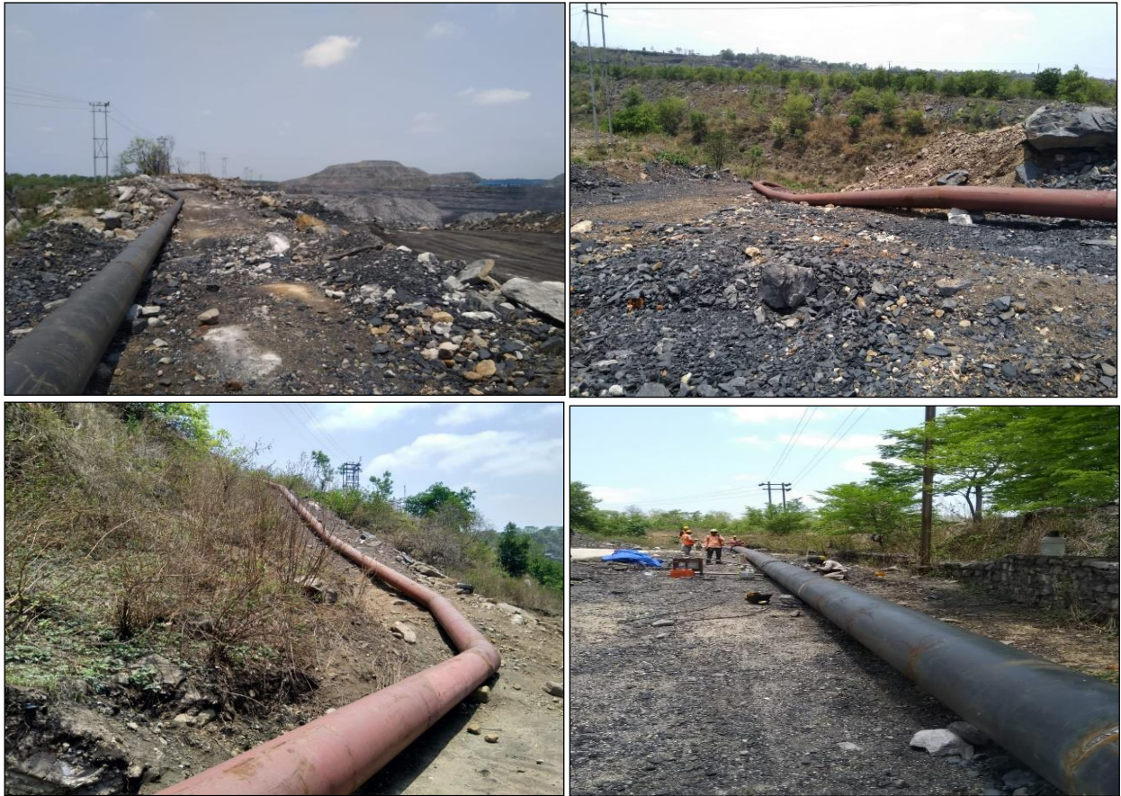
Pipeline installation from active quarry pit to abandoned mine pit
