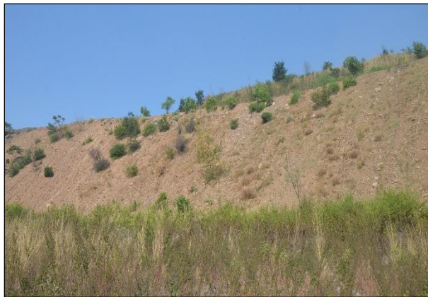
Soil & grass Spreading on dump slope
