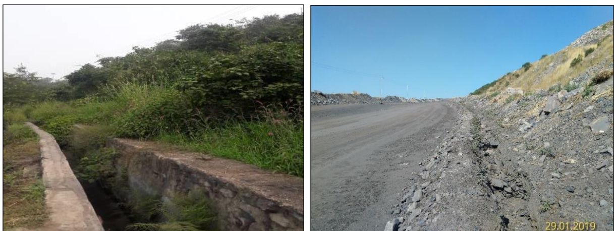
Catch Drains at the toe of dumps
