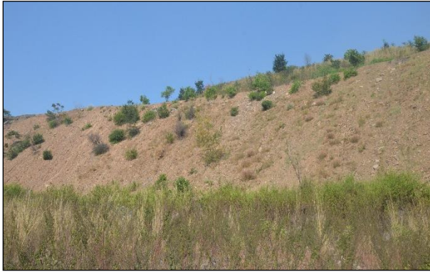
Top Soil spreading on dump for plantation
