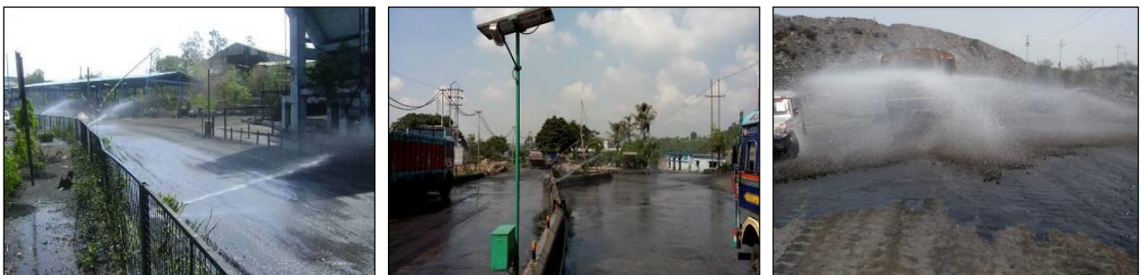
Use of fixed & mobile water sprinklers
