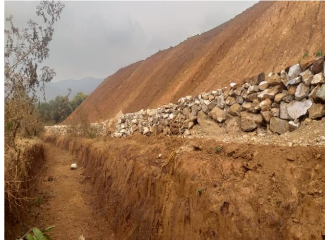
Dump runoff management
