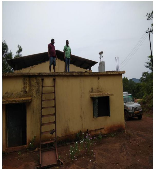
Air Monitoring Station
