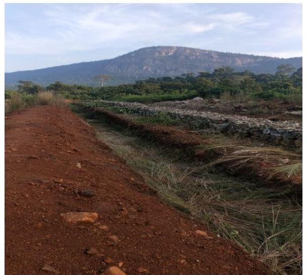
Garland drain with retaining wall cleaned
