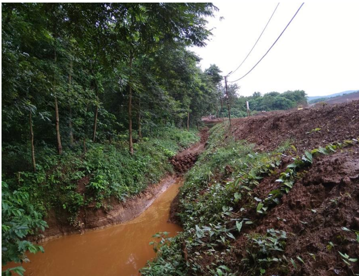
Garland drain with settling pin & Check dam
