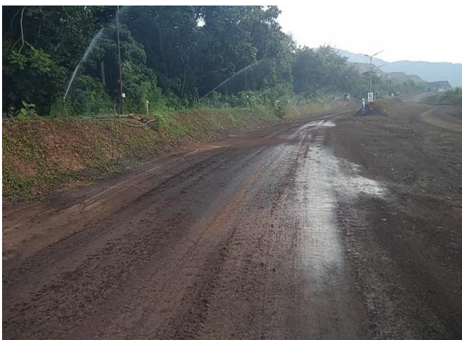
Mines haul road water sprinkling
