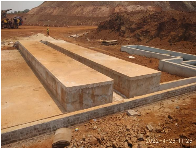
Vehicle washing with Oil & Grease separation pit
