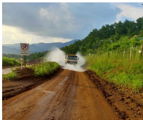
Water sprinkling through movable water tanker & Fixed Sprinkler
