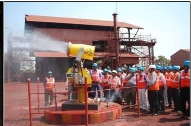
Water Mist System in Plant
