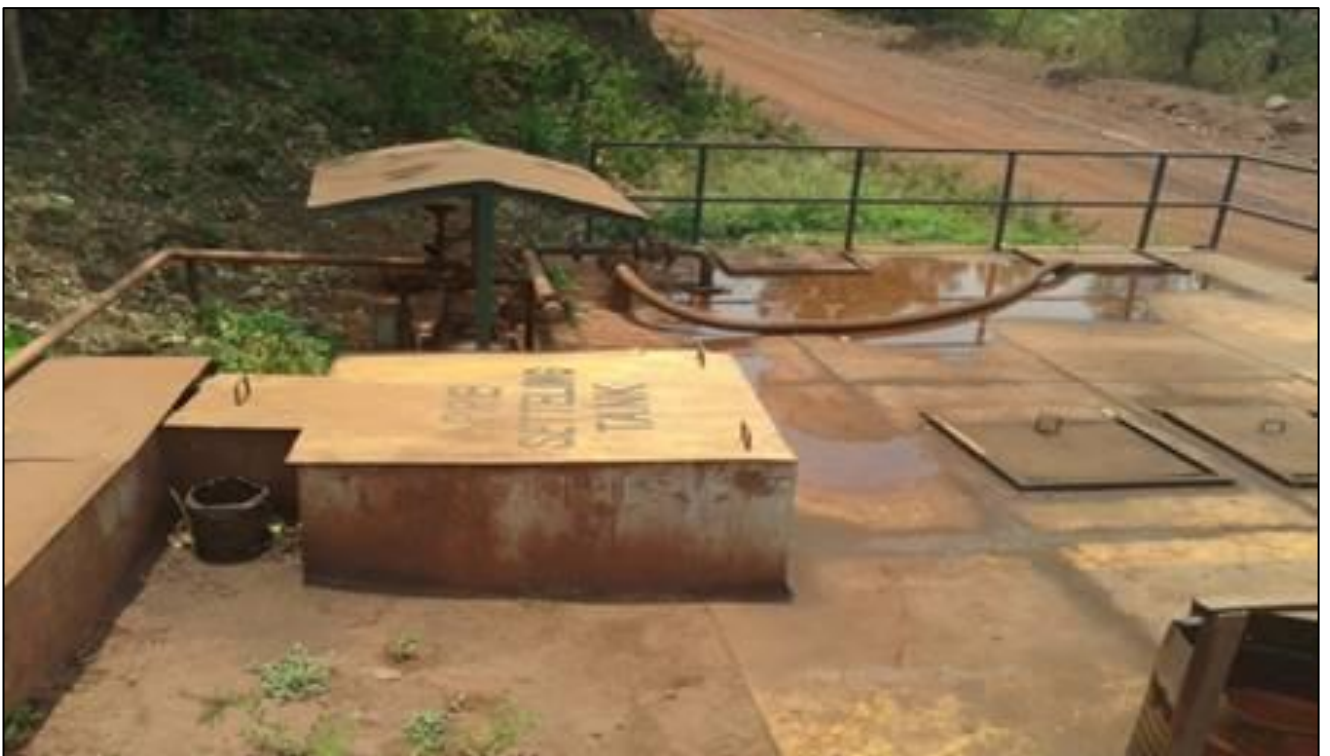
Oil & Grease Separation Pit
