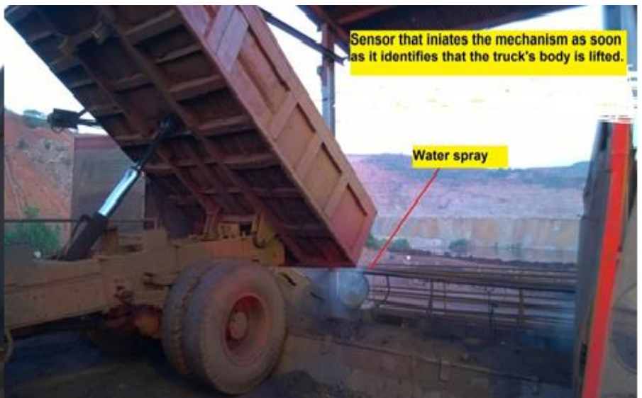
Dust Suppression System at Hopper
