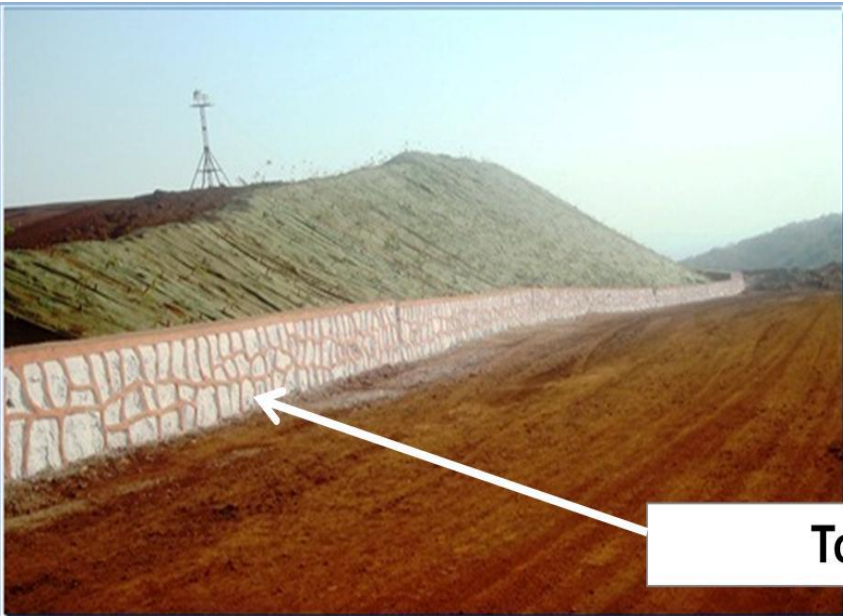
Toe Wall & garland drain
