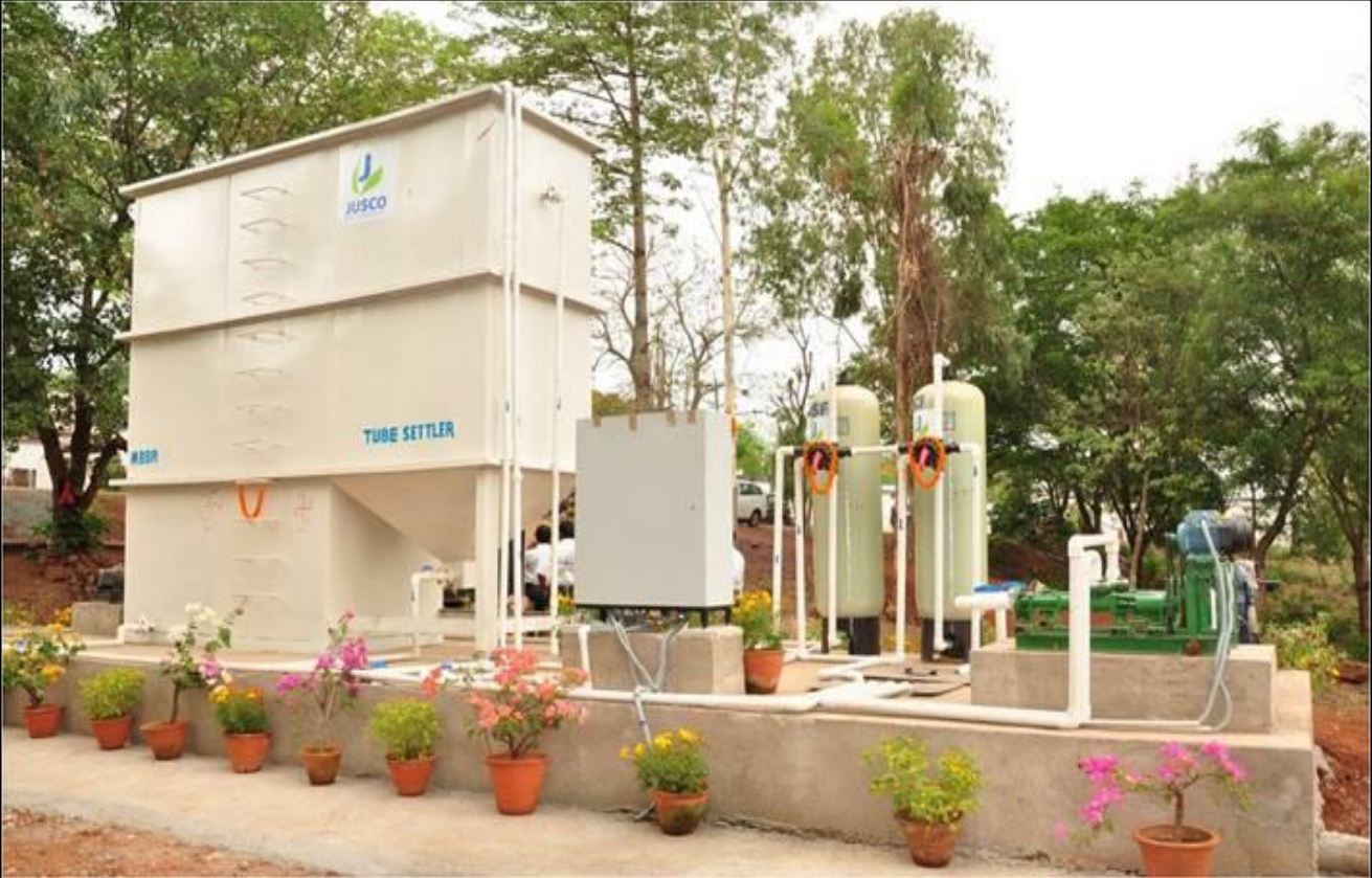
Sewage Treatment Plant
