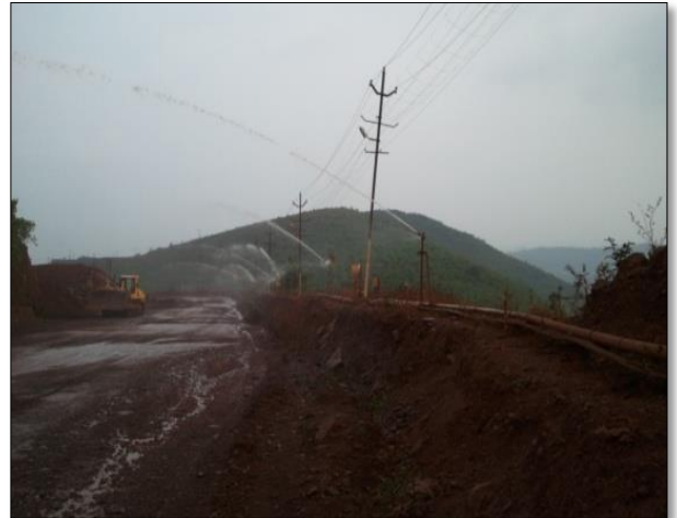
Stationary Water Sprinkler
