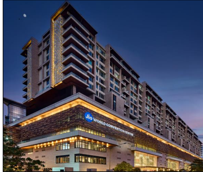
Tata Steel LRPC 1 strands used at Jio World Centre, Maharashtra
