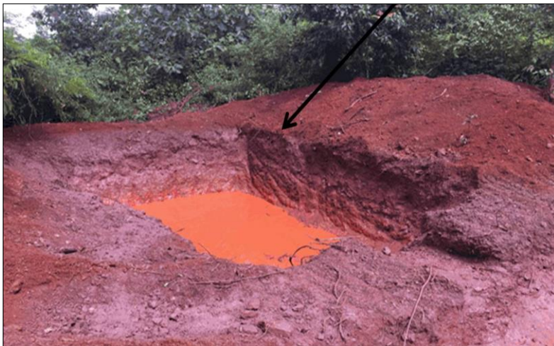
Settling Pit for Surface Runoff Management
