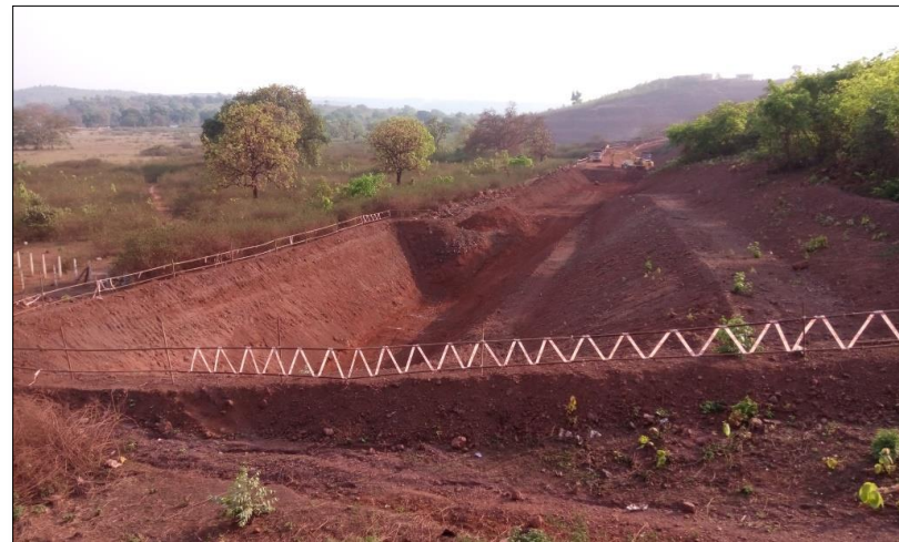
Settling Pit for Surface Runoff Management
