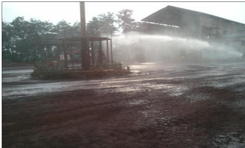
Fixed Water Sprinkler
