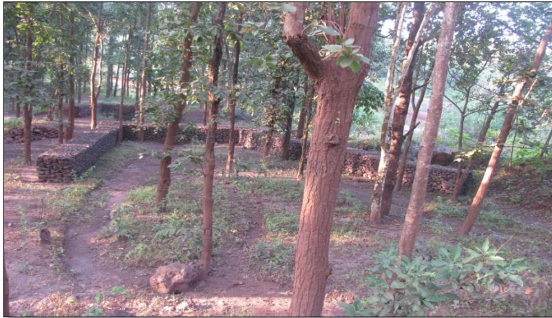
Check Dam for Surface Runoff Management
