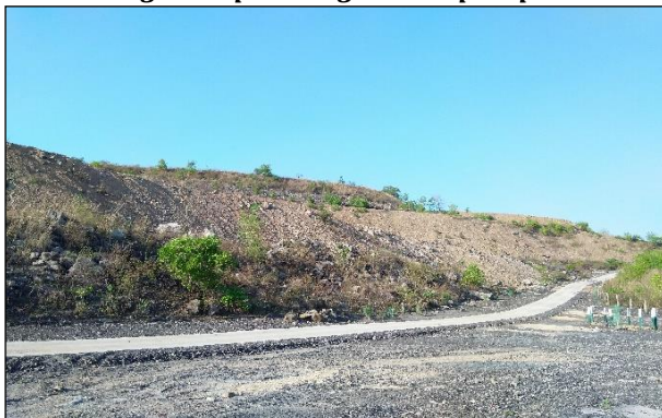
Soil & grass Spreading on dump slope
