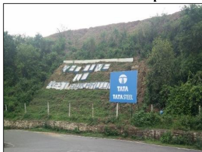
Toe walls on dumps
