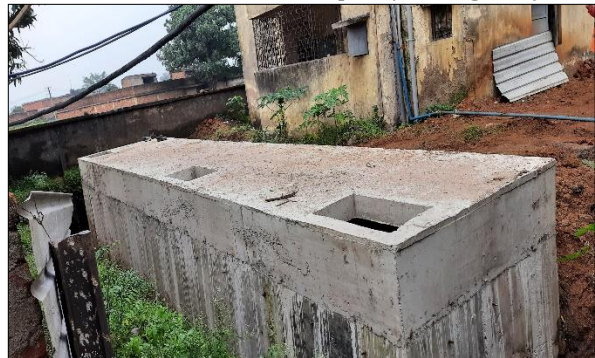
100 KLD STP at Chainpur (In Progress)
