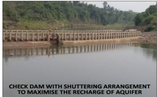
Check Dam to increase ground water recharge
