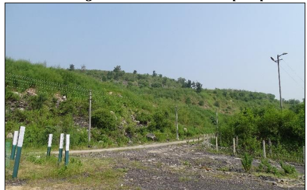
Grassing and Plantation on dump slope
