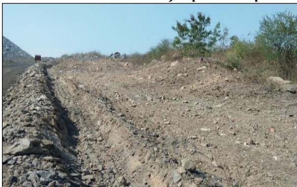
Maintained catch drain of Top Soil Dump
