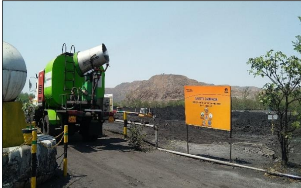
Water Mist Canon in coal stacking area
