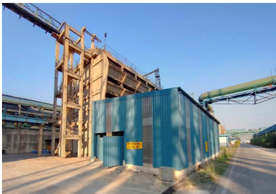
Hazardous Waste ( oil barrels) storage shed
