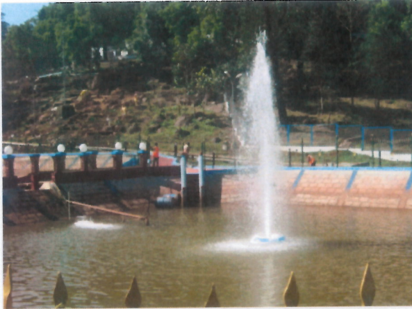
Rain water harvesting pond Noamundi
