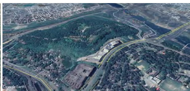
JMD after rehabilitation on October 2018
