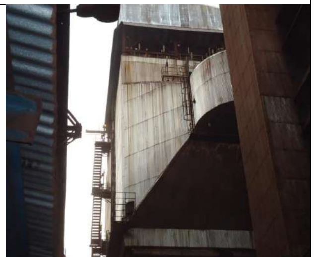
Sinter Plant 2 New Waste Gas ESP
