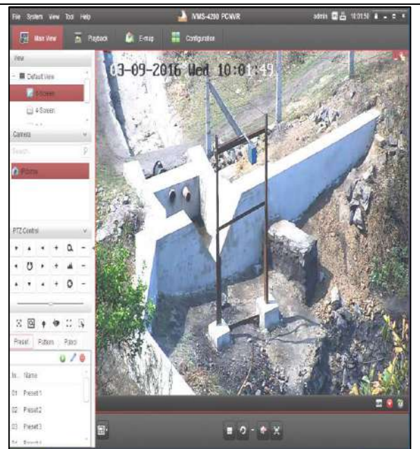
Effluent Analyzers & Monitoring
