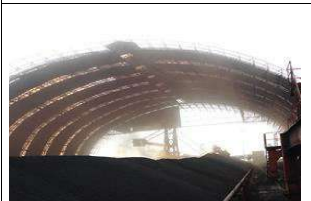
Covered Shed for Coal and Pellet
