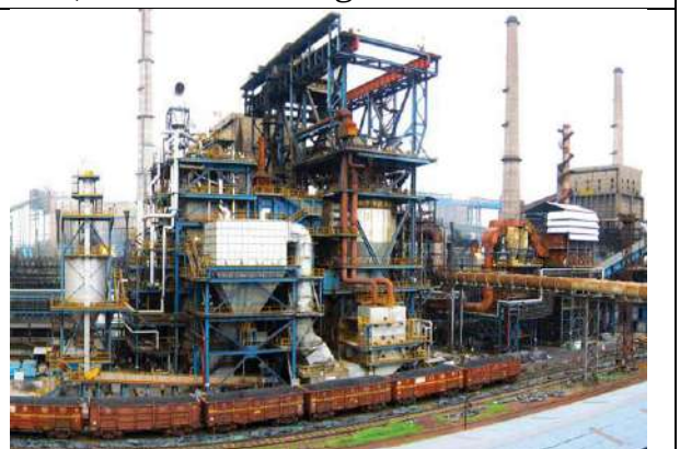
Waste Heat Recovery in Coke Dry Quenching
