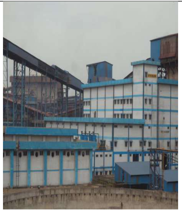
Reverse Osmosis Building
