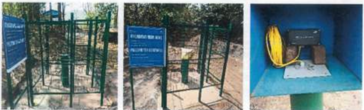
Piezometer (STP) with digital recorder
