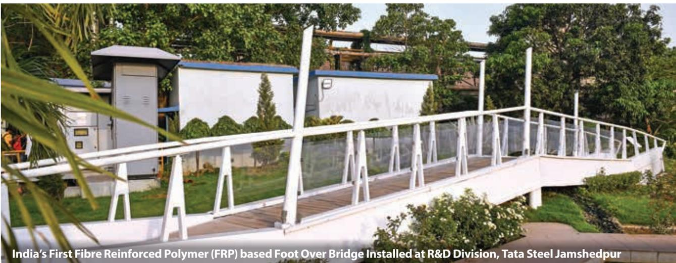
India's First Fibre Reinforced Polymer (FRP) based Foot Over Bridge Installed at R&D Division, Tata Steel Jamshedpur
