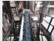
Sinter Plant, Wire & Rod Mill
