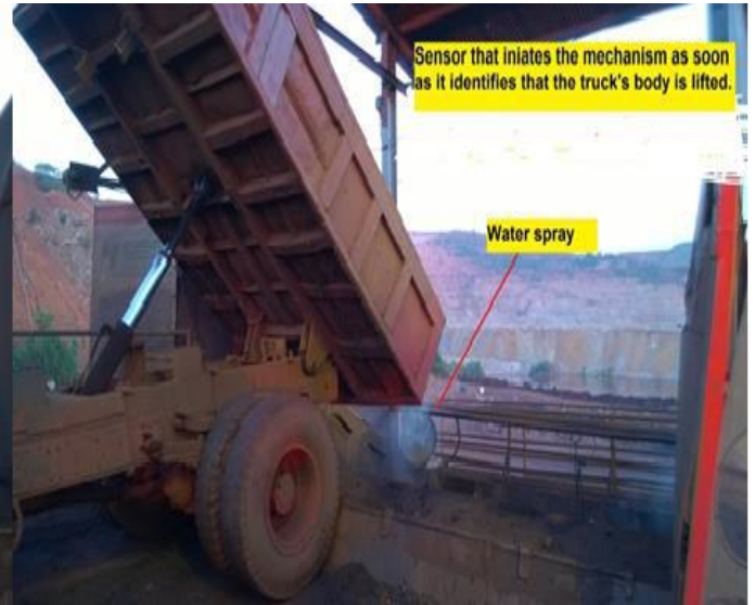
Dust Suppression System at Hopper
