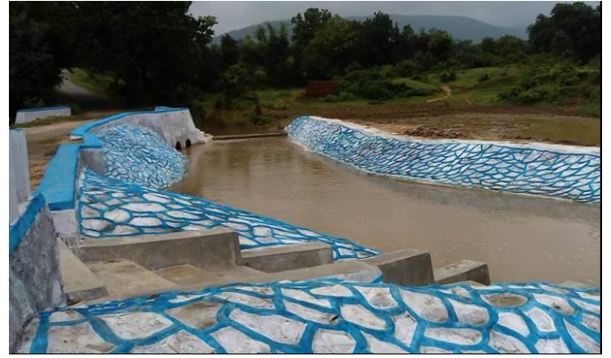
Check dam construction at Rahawan village
