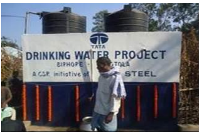
Drinking water facility at Birhore Tola
