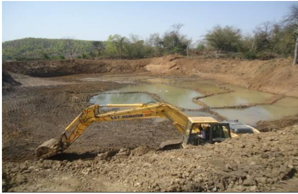
Rainwater Pond at Parsabera
