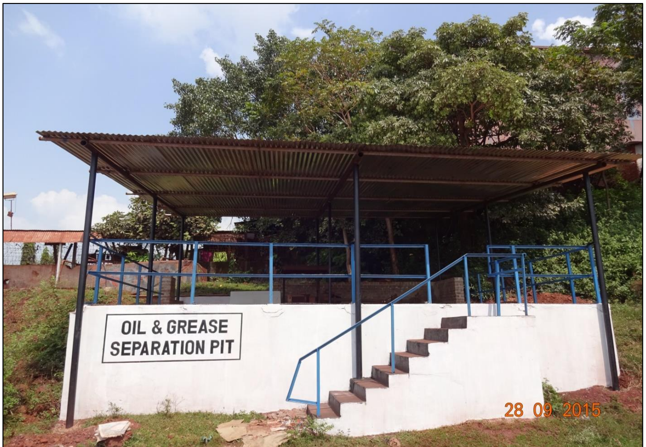
Oil & Grease Separation Pit
