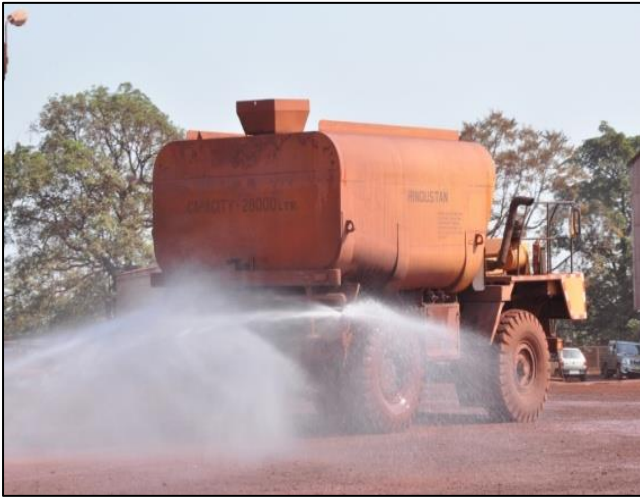
Mobile Water Sprinkling
