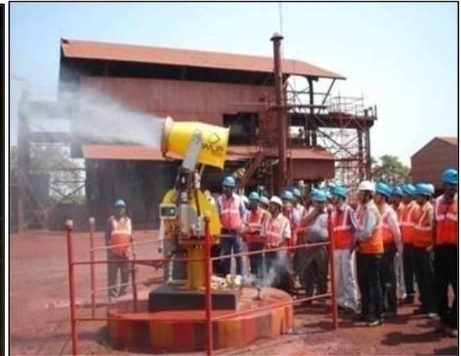
Water Mist System in Plant
