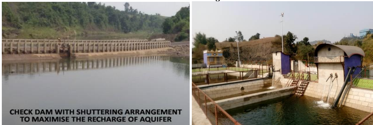
Check dam construction at Rahawan village
