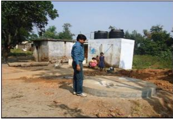
Artificial ground water recharge pit (Bore well) in Bilhore village
