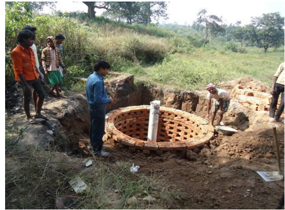
Artificial ground water recharge pit (Bore well) in Bilhore village
