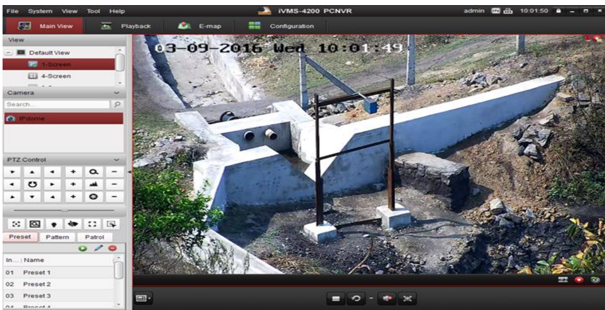
Live web camera footage installed at discharge point
