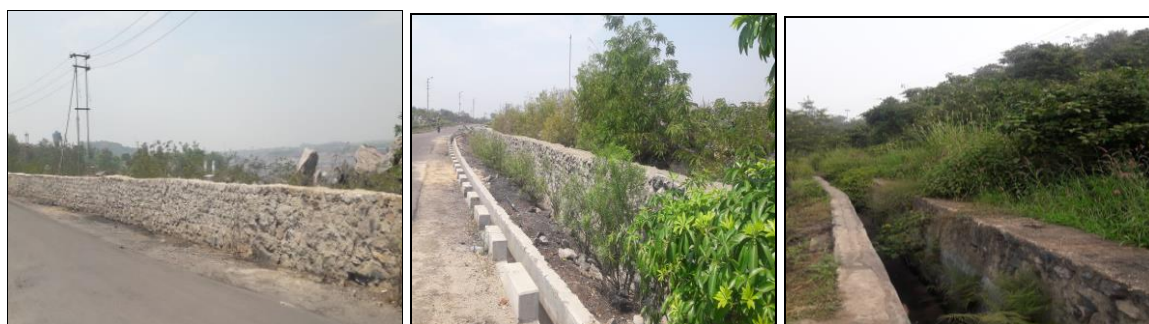
Toe wall & garland drain in the area
