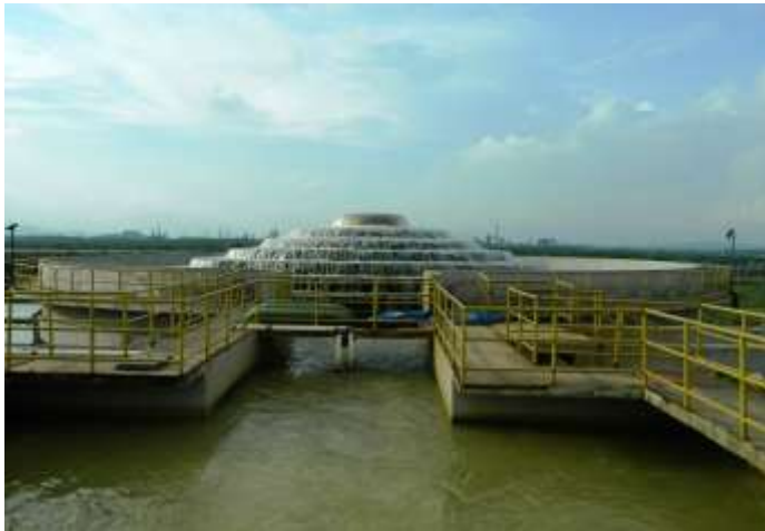
Cascade Aerator at Raw Water Treatment Plant
