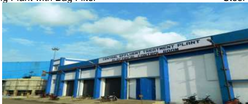
Central Effluent Treatment Plant
