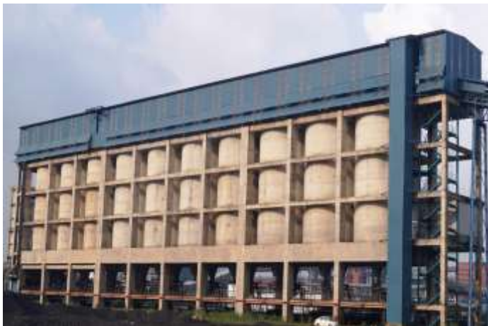
Coal blending bunker
