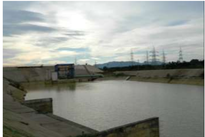
Storm water Reservoir
