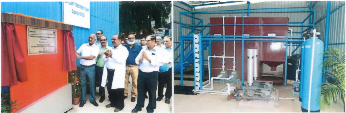
10KLD Effluent Treatment Plant (ETP) at Hospital
