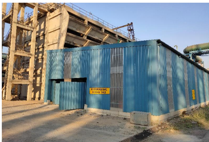
Used oil and Grease storage facility
