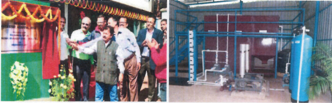
10 KLD Effluent Treatment Plant (ETP) at TATA Steel Hospital Joda (Dec 2017)
