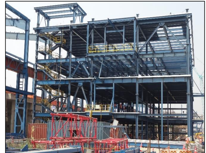
ECR Building of PLTCM
