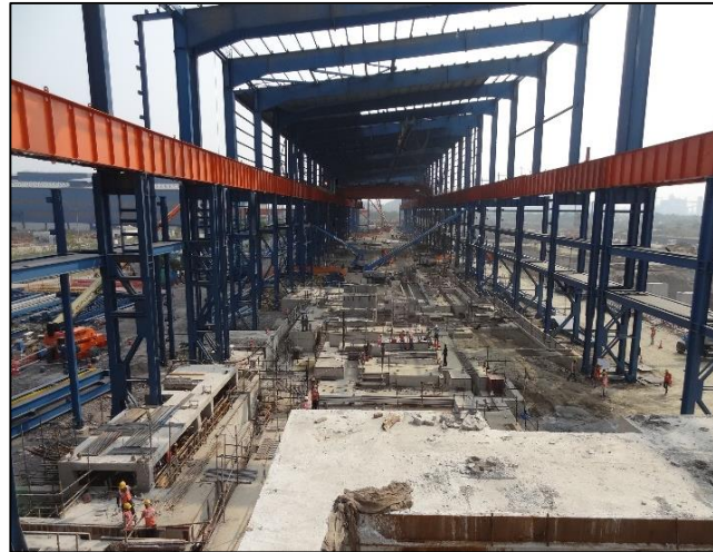
Entry side equipment foundation of PLTCM
