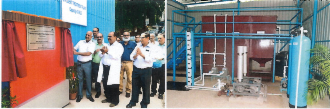
10 KLD Effluent Treatment Plant (ETP) at TATA Steel Hospital Noamundi
