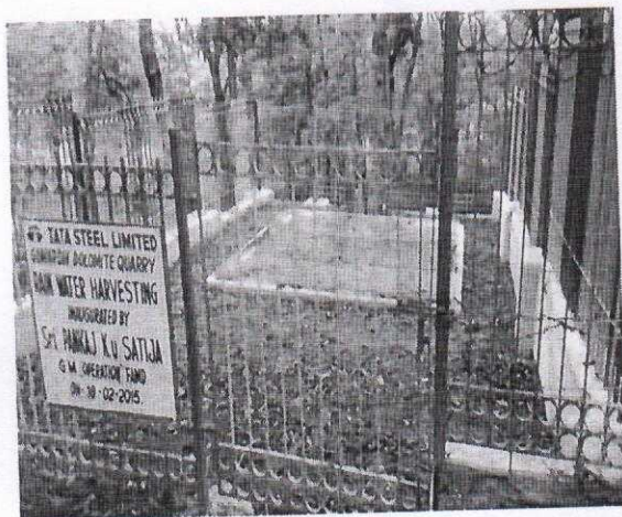
RECHARGE PIT OF ROOF TOP RAIN WATER HARVESTING STRUCTURE OF GUEST HOUSE OF GOMARDIH
