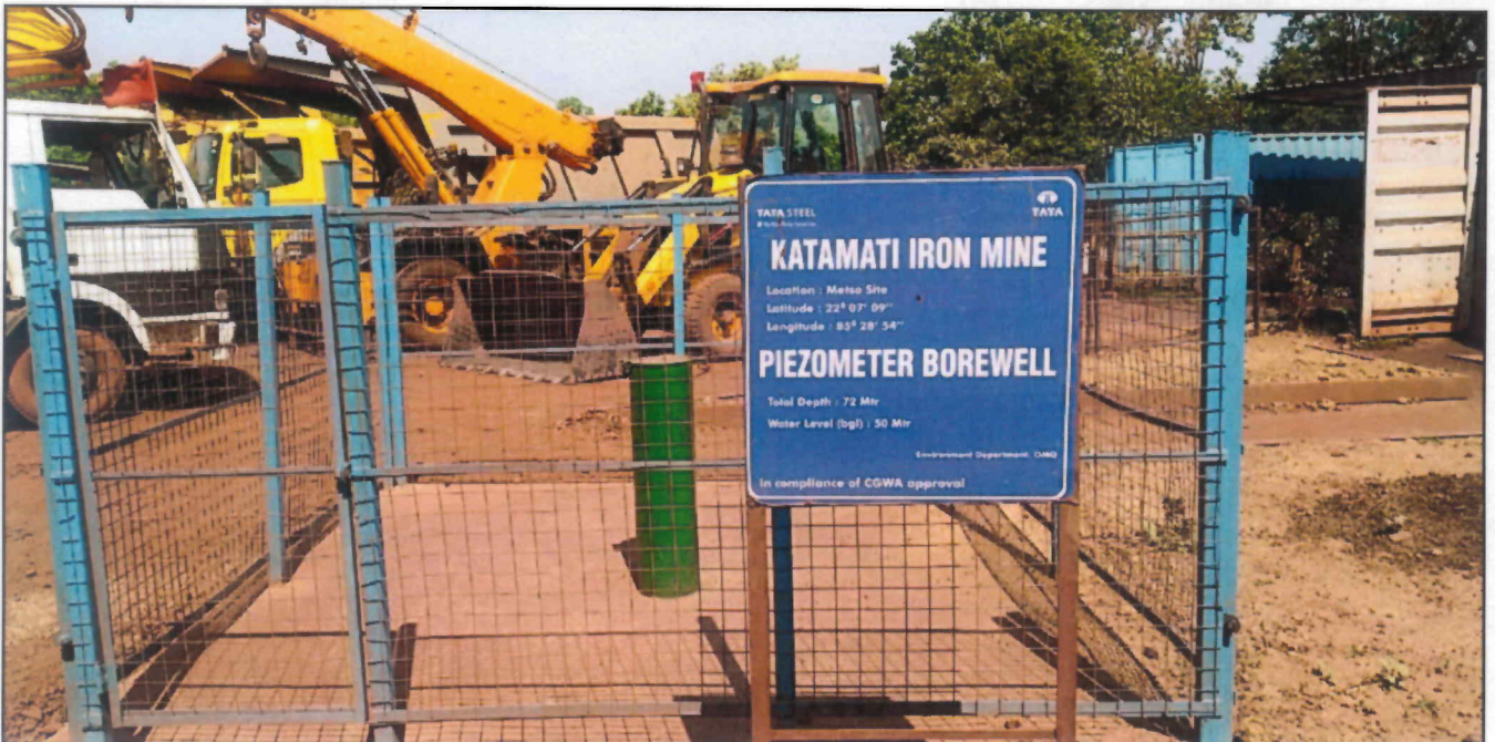
Piezometric borewell installed at METSO Office site, Katamati Mine
