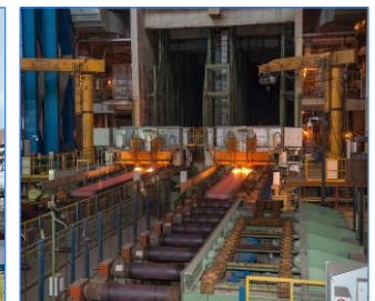
Steel Melting Shop
