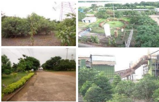
Concrete Road & Green Belt Development at Ferro-Chrome Plants
