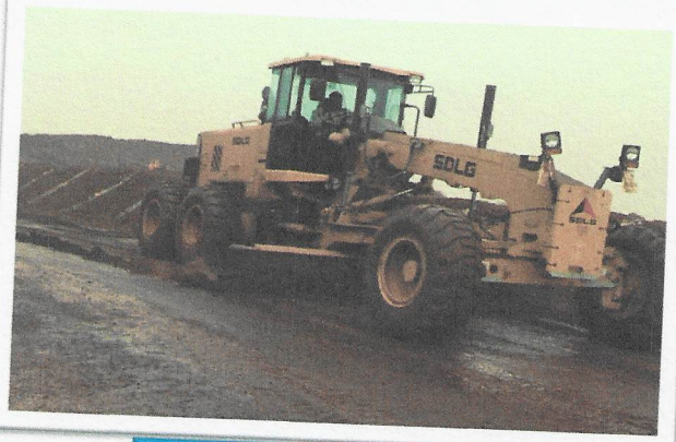
Grader for Haul Road
