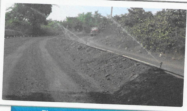
Fixed Sprinkling System
