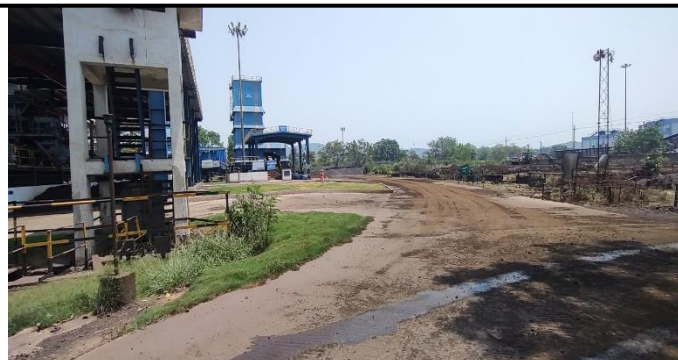
Newly constructed RCC roads
