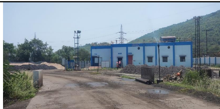
Newly constructed RCC roads and water sprinklers
