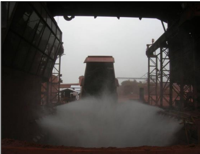
Water Jet System at Unloading Point
