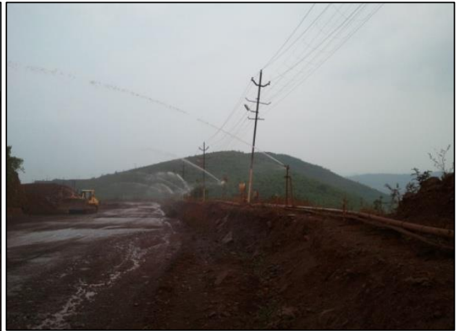
Fixed Water Sprinkler
