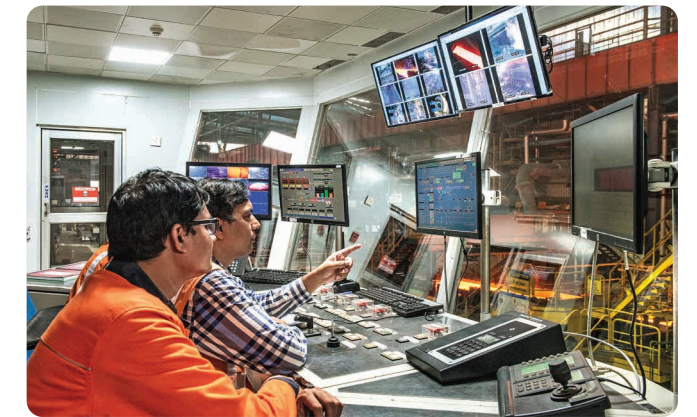
Control Room, Hot Strip Mill, Tata Steel Kalinganagar Works
