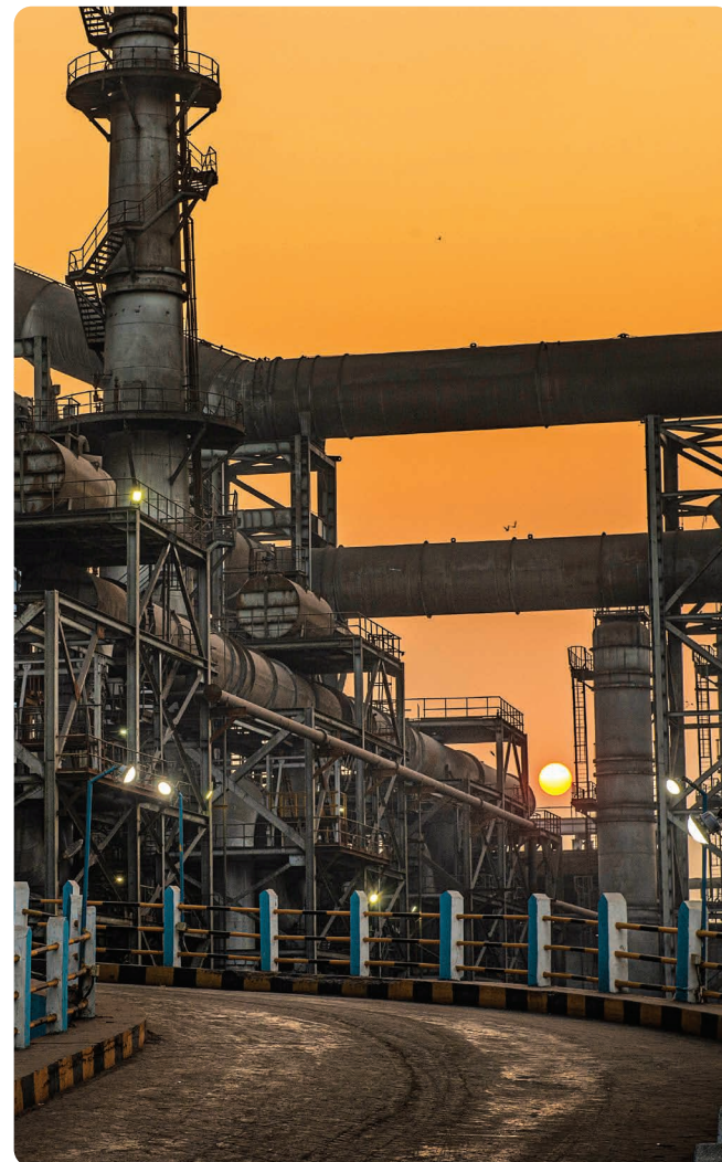
Blast Furnace, Tata Steel Meramandali Works
