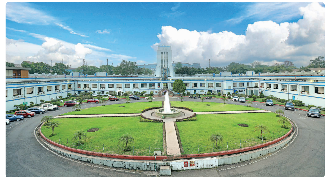
R&D building, Tata Steel Jamshedpur Works
