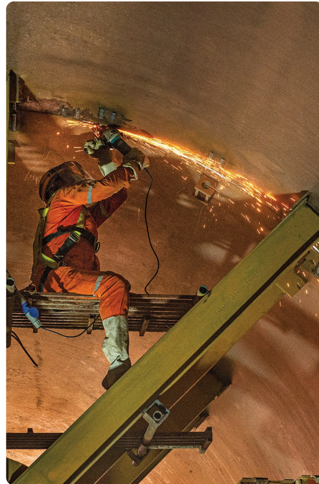
Blast Furnace, Tata Steel Kalinganagar Works
