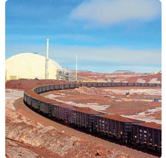
Rail Loop, Tata Steel Minerals Canada
