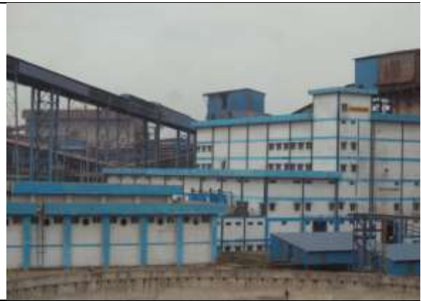
Reverse Osmosis Building
